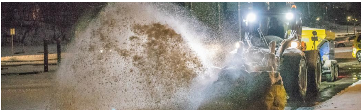
A sweep-salting measure on a bicycle path in Stockholm when a large amount of salt is swept off the surface.
