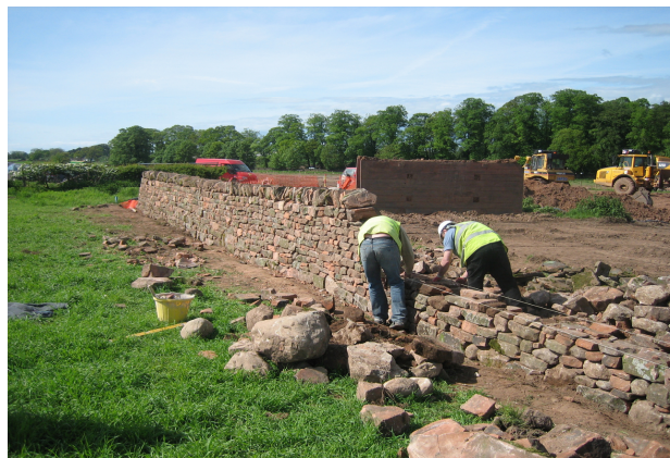
Above: River Eden Bridge under construction Below: Dry stone walling
