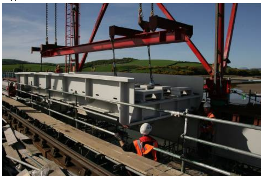
Above: Bespoke lifting gantry installing new battledeck type deck unit.
