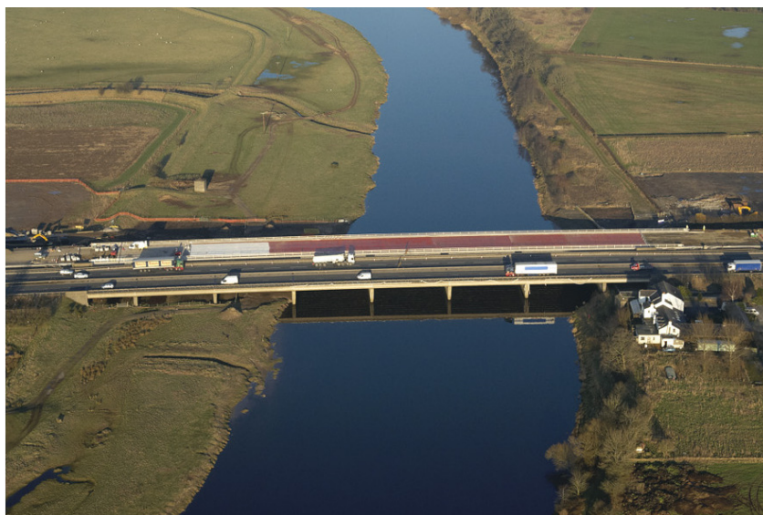
Above: New bridge crossing the River Esk; the third new crossing since Telford's original 'metal bridge' in 1815
