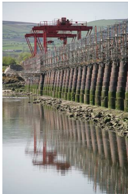
Above: Two lifting gantries were key to delivery in half the original timescale
