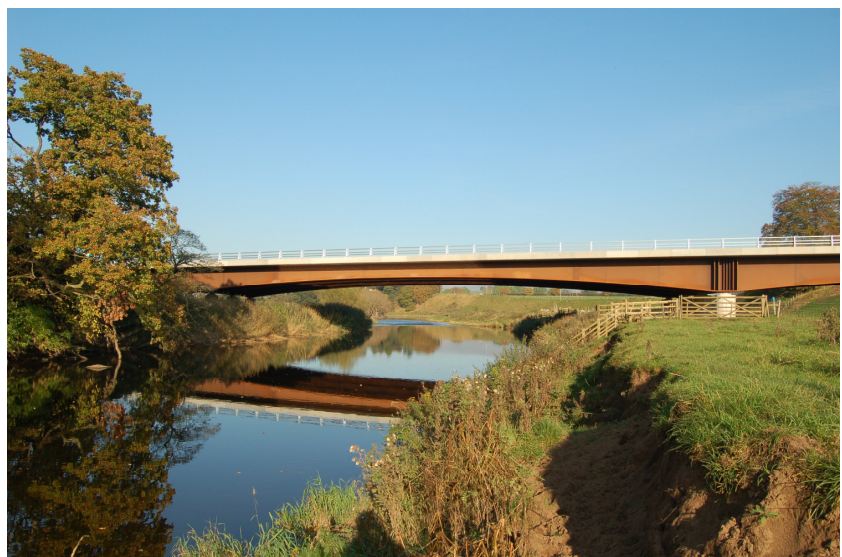
Above: River Eden Bridge
