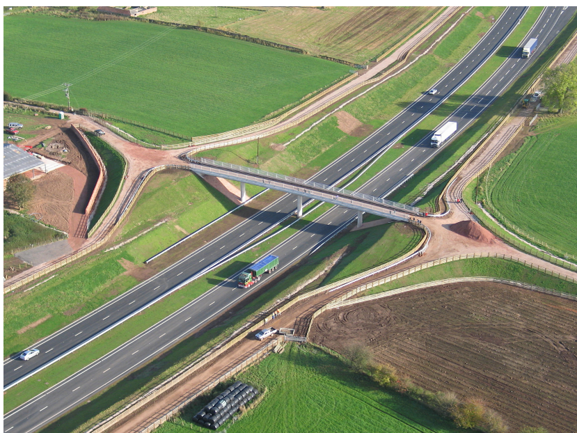
Above: Acton Lodge Bridge
