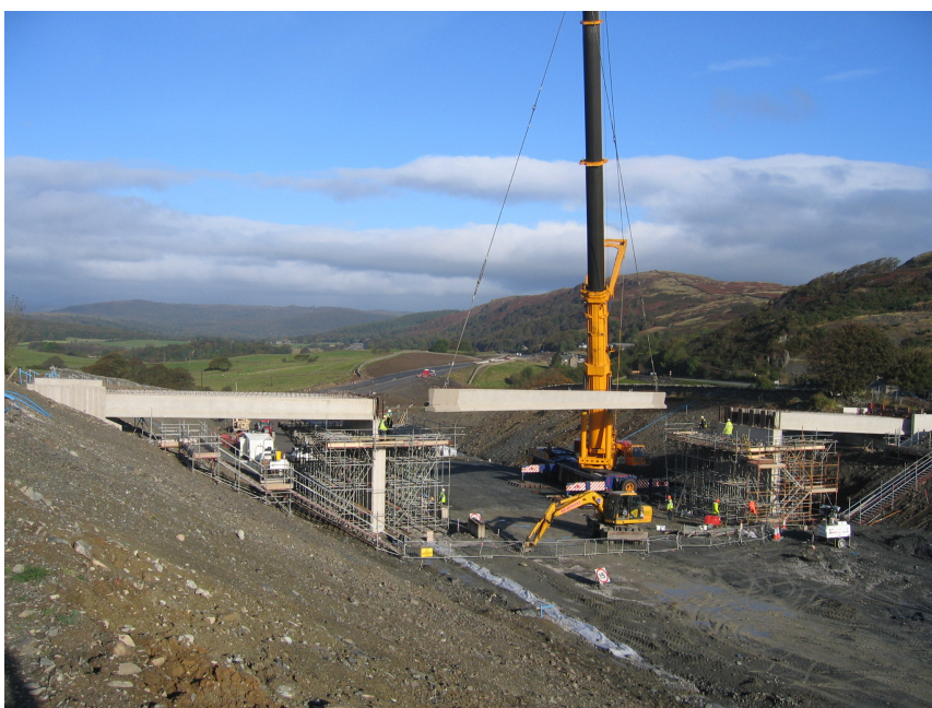
Above: One reinforced concrete overbridge and four underpasses have been constructed.
