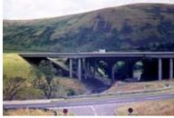
The 82ft [25m] high Borrowbeck viaduct is close to and 10 ft. higher than the stone arch railway viaduct carrying the West Coast main line, with the central span designed to frame the railway viaduct when viewed from the realigned A685. It was of great interest to us that a tall stone viaduct, constructed in 1850 for what were then, relatively light trains travelling slowly, now had huge Deltic diesels pounding over it at up to 90mph, apparently with no ill effects to the structure.
